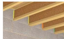
No mortar or mastic required to internal face. Hi-Vis Grippers visible for post installation inspection prior to plasterboard being installed.
