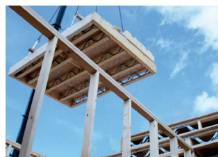
SpaceJoist and SpaceRafter cassettes can be delivered to site and craned into position to save build time.
